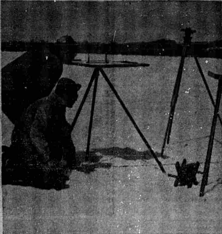
Conservation Department surveyors are kept busy during the winter collecting data from inland lakes in Michigan. Bottom contours, lake depths and outlines, weed beds and shore line features are among the major items surveyed. They are later charted on maps to aid the Department in its fisheries research and management programs. The maps also serve as excellent guides for fishermen.
